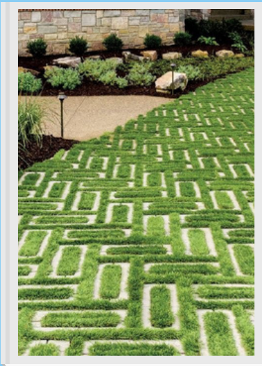
Grass pavers turn an impermeable surface into a permeable one
