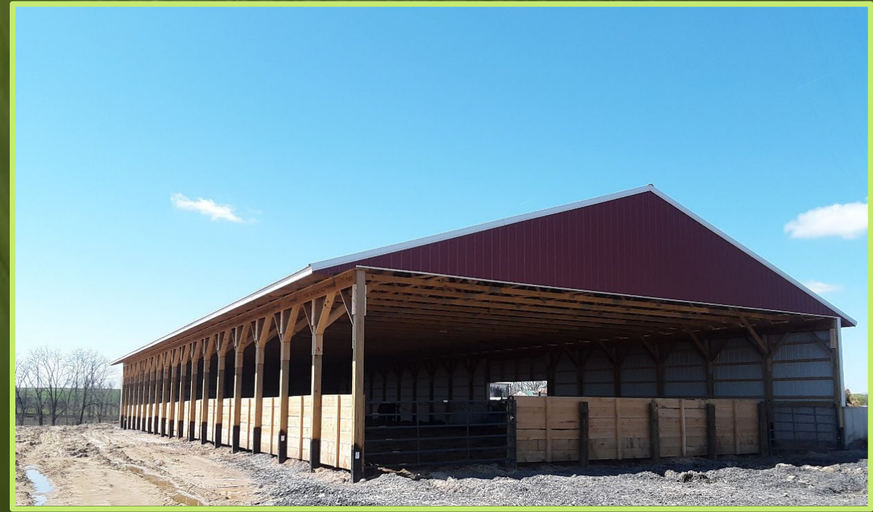
1 - Covered Barnyard for Heavy Use Area Runoff Management System
